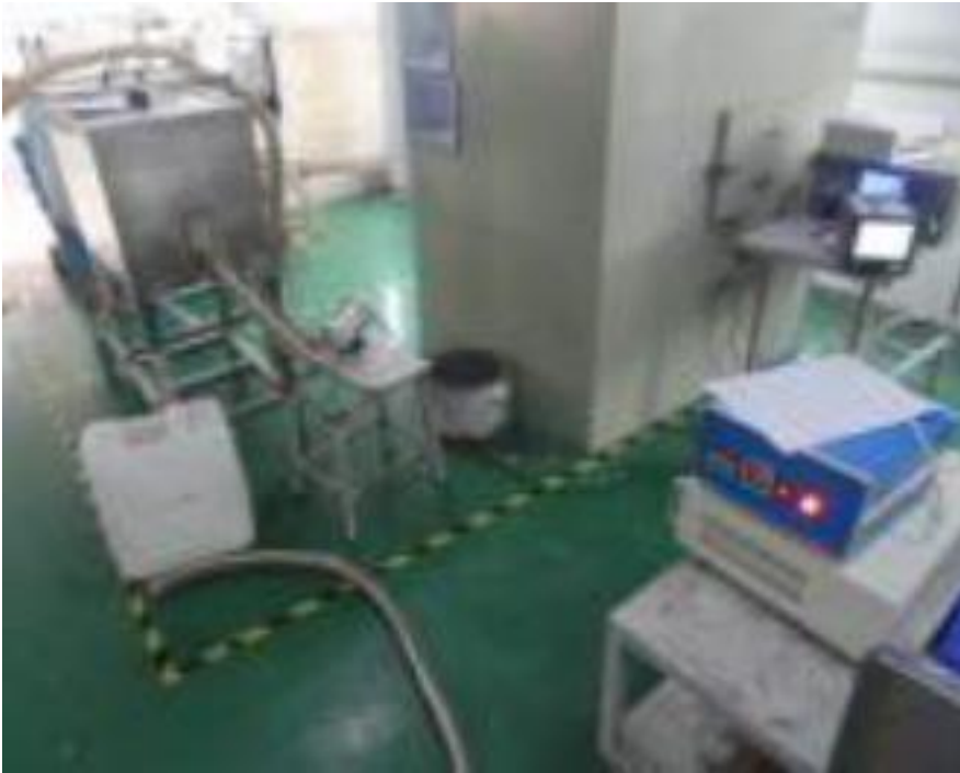
DC Power Test Tank
